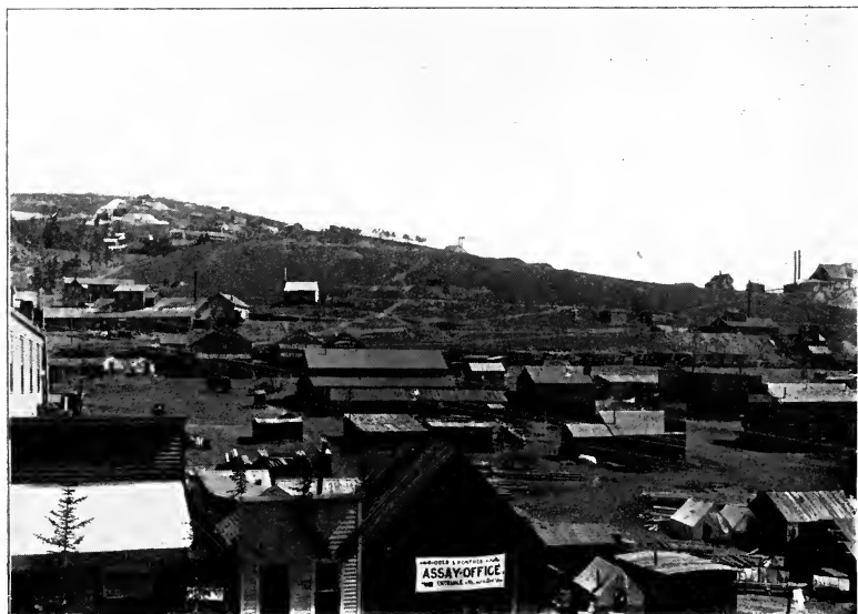
FIG. 110.—View of Battle Mountain, Victor, Colorado. From a window in Victor. The Portland group of mines is on the left in the background. The Independence mine is on the extreme right. From a photograph by J. F. Kemp, July, 1895.
